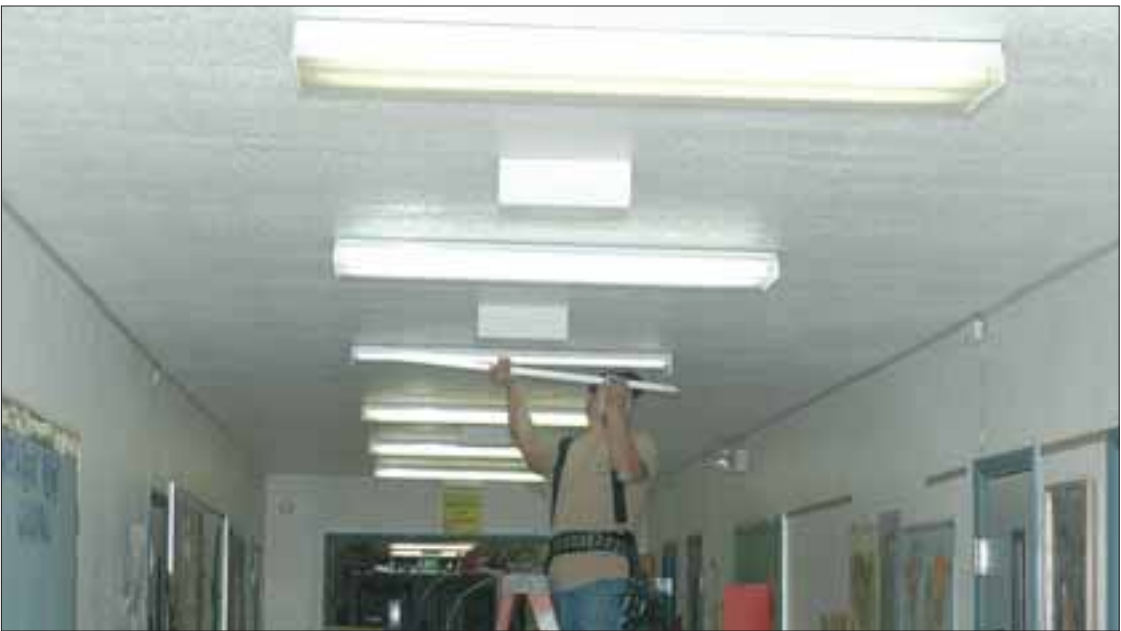
Softer, more efficient lighting installed Fabian Luna of Bender Electric snaps in a new fluorescent bulb in a Homedale Elementary School hallway light fixture Thursday. The newer lighting is white; the older bulbs (foreground) give off yellow light.
